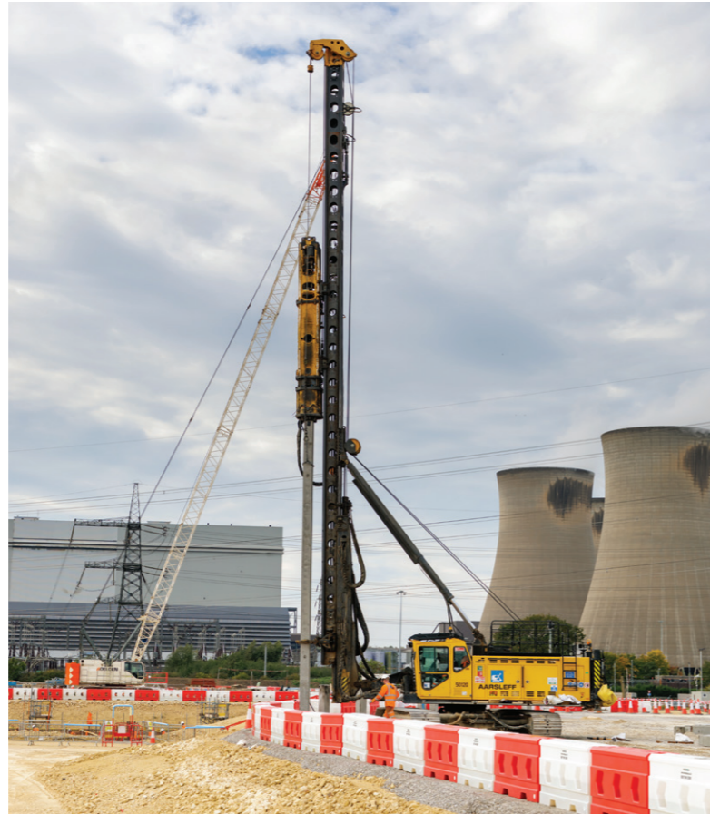
One of the piling rigs in use at Wren Hall Converter Station
