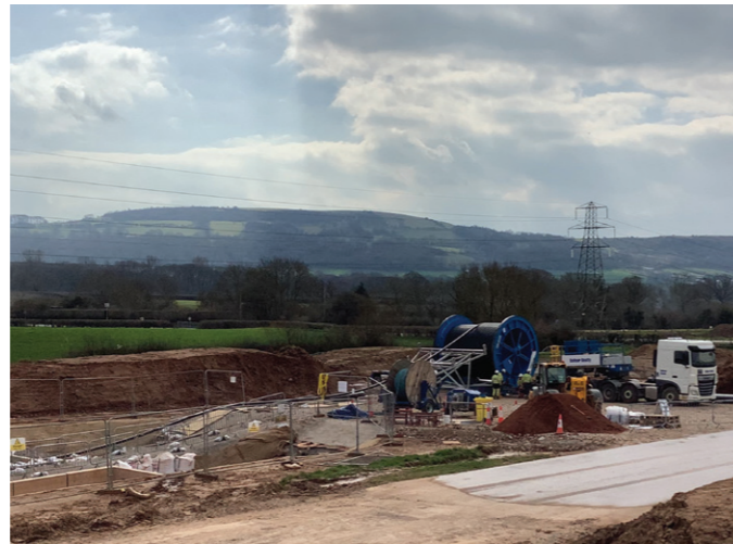
The ducted method of cable laying
