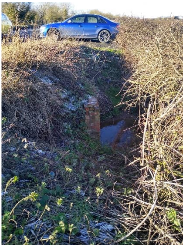
Photo 3 – Ditch and Brick Headwall to Culvert
