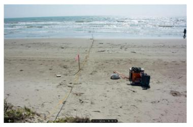
The work will involve the use of handheld probes and cable to gather detailed information that will inform our design for the landfall construction of the marine cable project.
